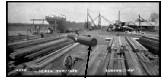
This photo shows the boilers used under deck for hoisting sails and the anchor, along with numerous large timbers waiting to be put to use on a new barge. Note the large stiff leg derricks in the background and the smokestack from the blacksmith shop.
