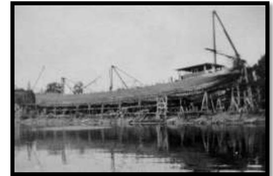
Photo of a barge nearing completion, with the scaffolding in place and the ways in the foreground. Average time of construction was approximately four months and employees worked year round, rain or snow.
